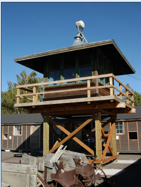
Guard Tower & Barrack, Tulelake-Butte Valley Fairgrounds Museum (Courtesy Kiyoshi Ina)
